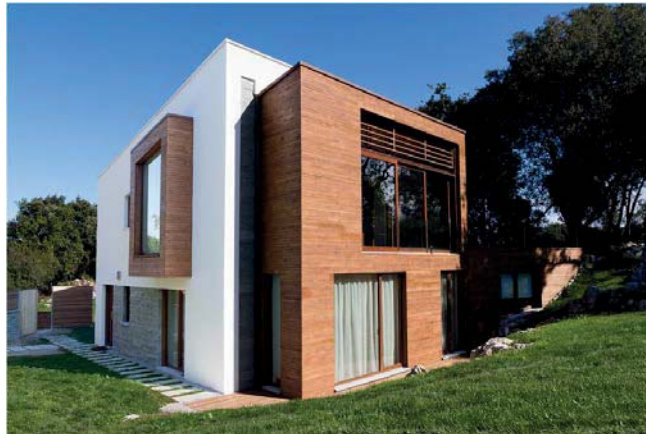
Figure 1: View of thermally modified Radiata Pine wood elements in a passive house.
