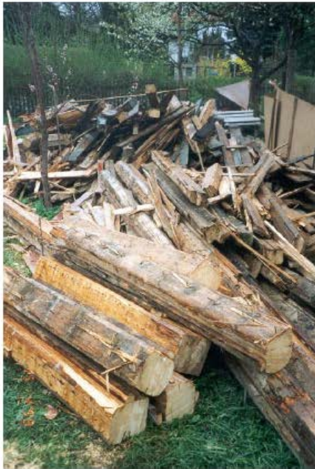
Construction wood waste from a controlled demolition process Picture by INTECUS
