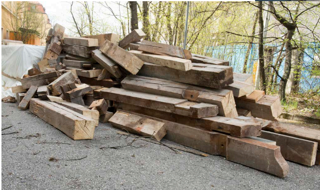
Selected dismantling of construction wood
