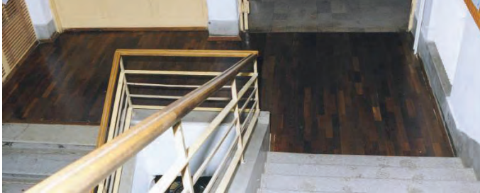
Figure 1: The appearance of the floor after installation.
