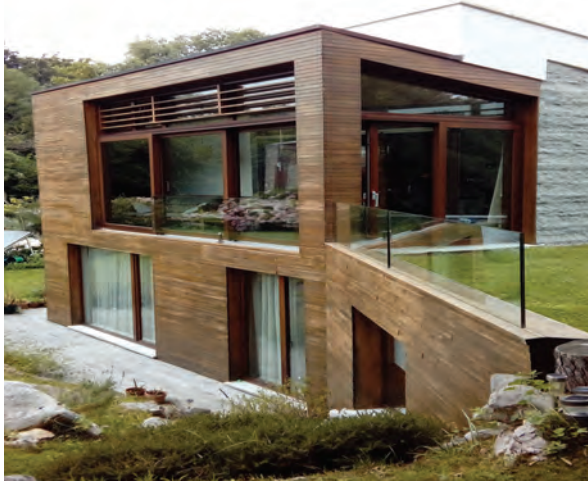
Figure 1: View of thermally modified radiata pine wood elements in a passive house.
