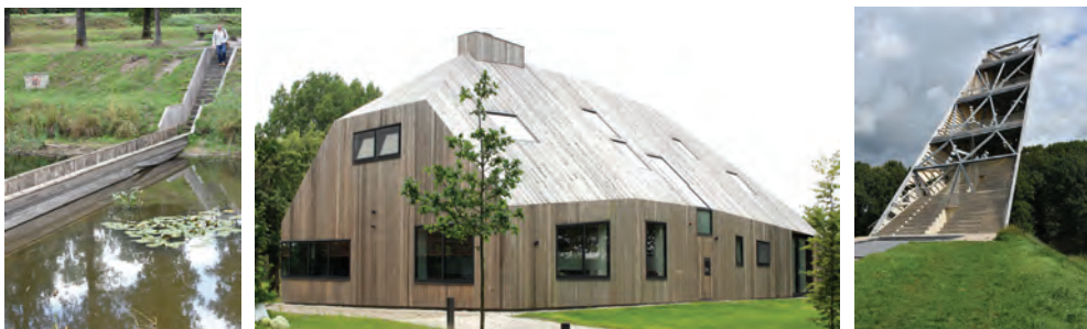
Figure 3: Examples of modified wood in construction, from the left: a) The Moses Bridge of acetylated wood in Fort De Roovere, the Netherlands, b) façade of thermally modified timber, private house in the Netherlands, and c) Outlook tower of acetylated timber in Fort De Roovere.
